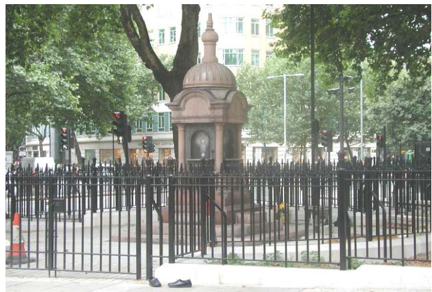
The new fenced and gated site.
