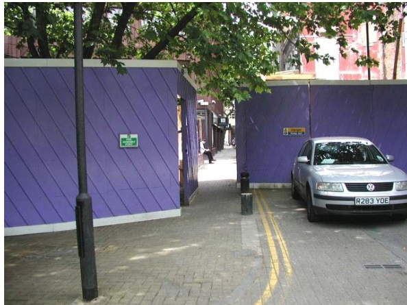
Let's hide the site office behind this hoarding and while we are at it create a nice obscured pathway.
