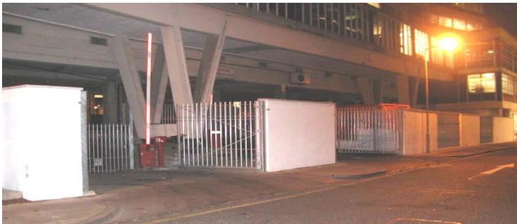
Now has full height, street level gates.
