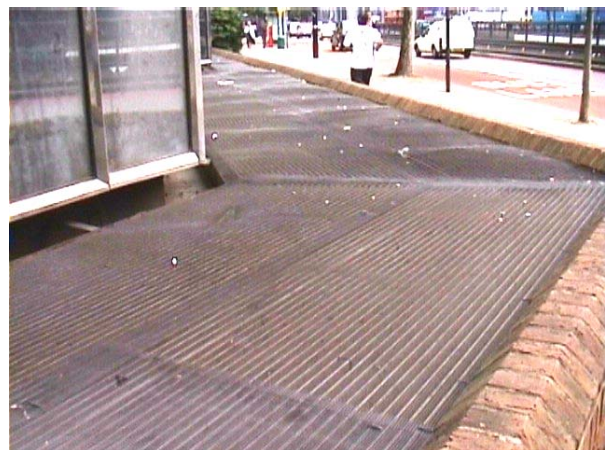
Fig 53: Mesh 'lid' with litter deposited on it.
