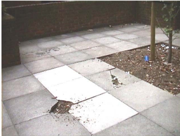
Fig 80: Broken paving slabs.
