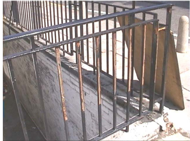
Fig 32: The poor state of the railings' repair.
