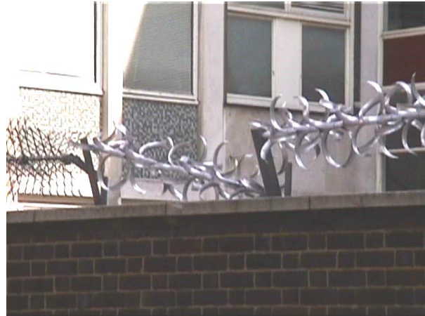
Fig 44: (Broken) anti-climb cacti.
