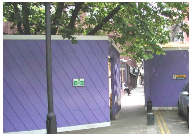
The diagonal battens successfully prevent fly posting. However, the hoarding around these site offices for a development nearby have greatly reduced surveillance of the street and into the site.
