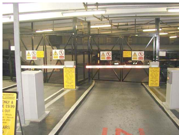
This vehicle entrance to Bloomsbury Square underground car park includes booms and floor to ceiling security gates. The staffed office is out of picture to the left.
