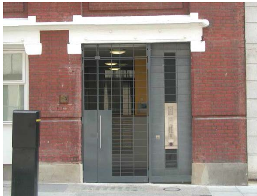
This entrance door to a block of residential flats in King's Cross opens inwards and is therefore flush with the building line
