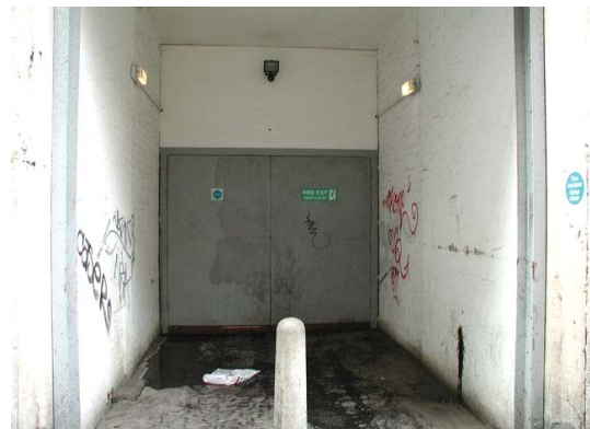
This deeply recessed door shows evidence of all types of misuse from rough sleeping and drug use to graffiti – some of which is in blood. Note too the bollard, which is intended to stop motor vehicles from blocking the exit.
