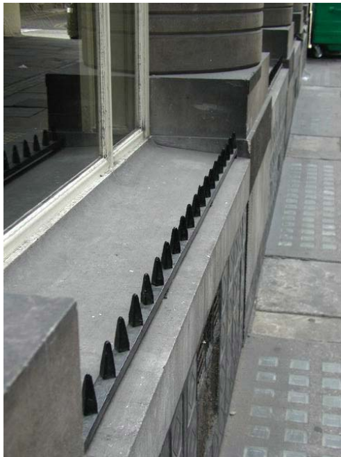
Serrated blade on a low wall outside a fast food restaurant.
