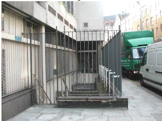
This 2.2m railing and gate around a light well at the back of an office building have prevented the return of the drug users. A fine steel mesh prevents public side access to the release handle on the back of the gate
