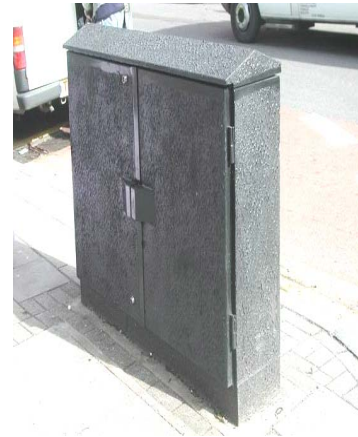
Stipple painted telephone cable cabinet
