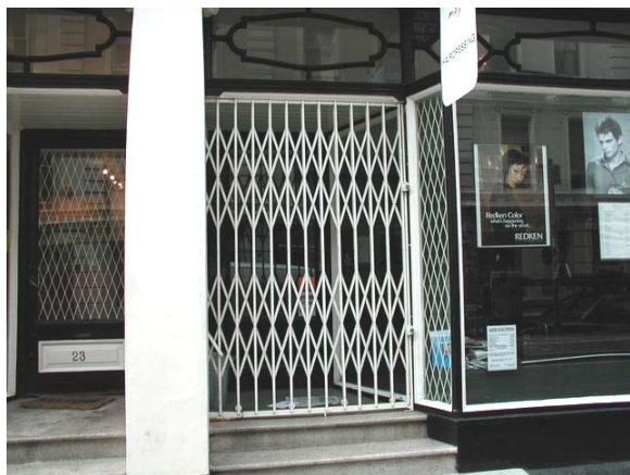
This shopkeeper pulls across and locks this concertina grille each night to protect the recess.
