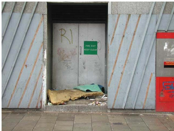
These recessed emergency exit doors were brought forward (see right) as the building they serve currently stands empty awaiting redevelopment
