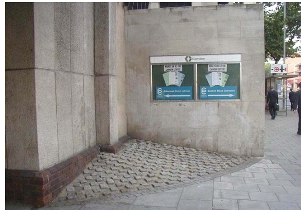
The bench was removed and the small concrete blocks set into sloping concrete have successfully deterred loitering
