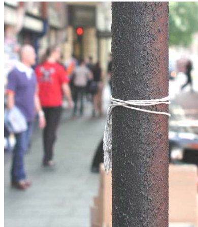
The stippled paint has forced the advertiser to tie the advertisement around the pole. This is less damaging and easy to remove.
