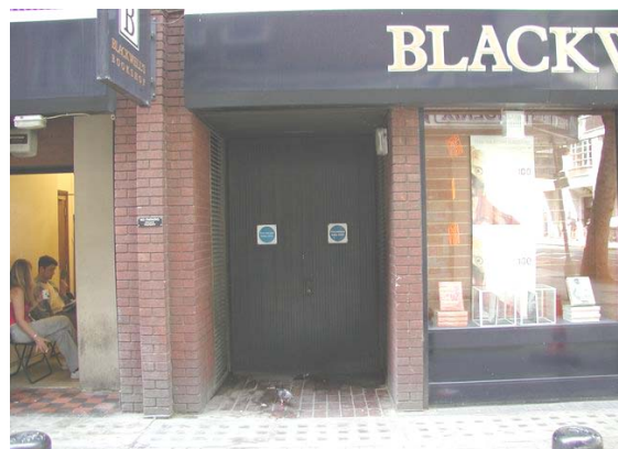
The private forecourt in front of these doors could enable these emergency exit doors to be brought forward.
