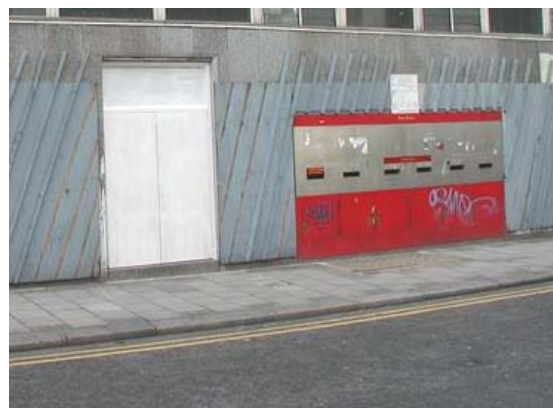
These recessed emergency exit doors were brought forward (see right) as the building they serve currently stands empty awaiting redevelopment
