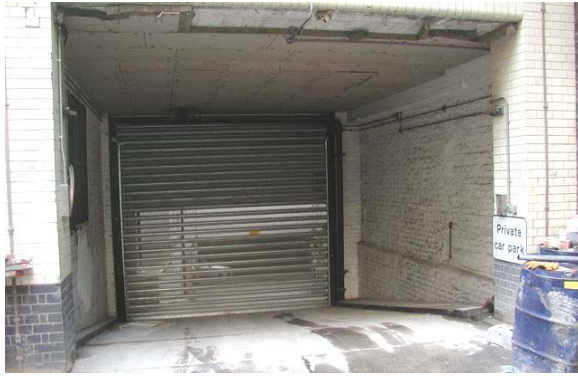
A poor example of an entrance to a private underground car park, which creates a large and unmanageable recess.
